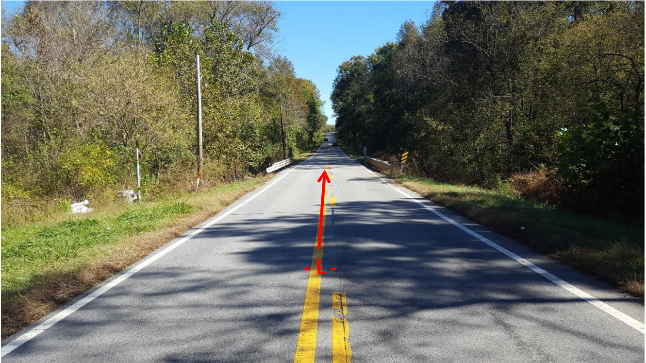
Photograph No. 1: View looking towards EB1 to EB2
