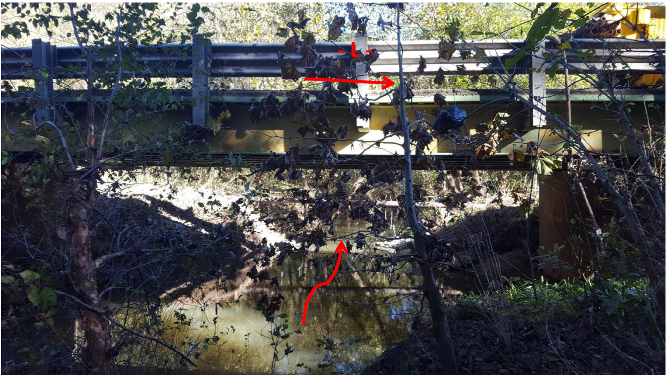
Photograph No. 2: View facing downstream.
